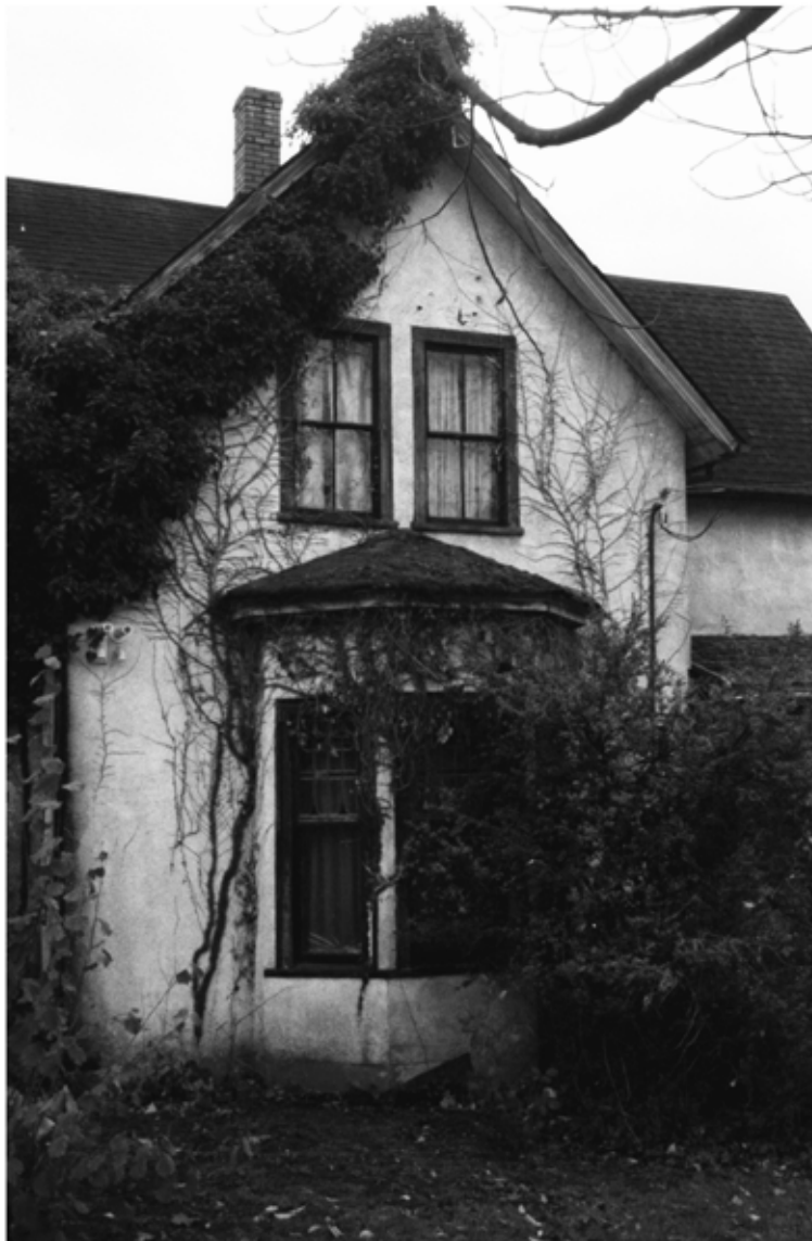
04. Shot on near infrared Washi Z film, this abandoned home slowly decays, a fine example of colonial opulence from bygone halcyon days. Consumed and turned to inevitable rot by vine, creeper and mould. • Kyle Mason
